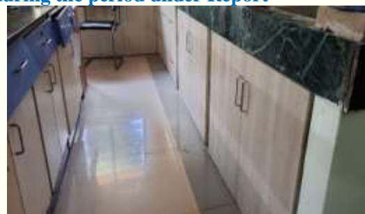
Renovation of UG laboratory at Veterinary College, Navsari
