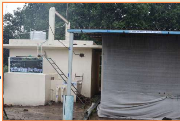
Roof top rain water harvesting
