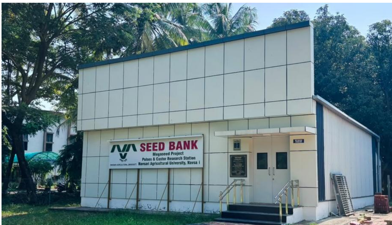
Seed Bank Facility Established Under RKVY
