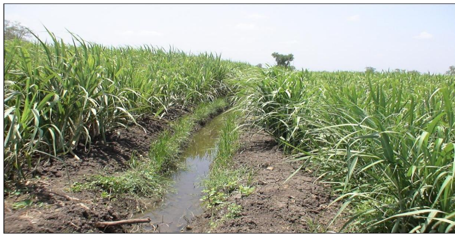
Digging of open drain
