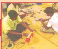
Sealing of blocks
