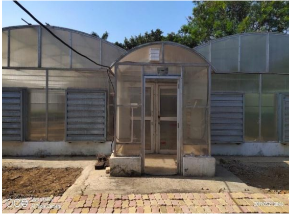
Green House (Polycarbonate with automatic fogging and cooling facility)
