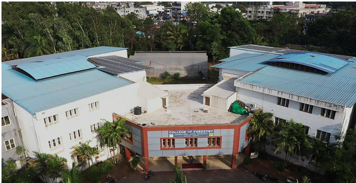
A view of premises of College of Forestry as Green Building with greenery by trees, solar energy systems, rain water harvesting system & ground water recharge
