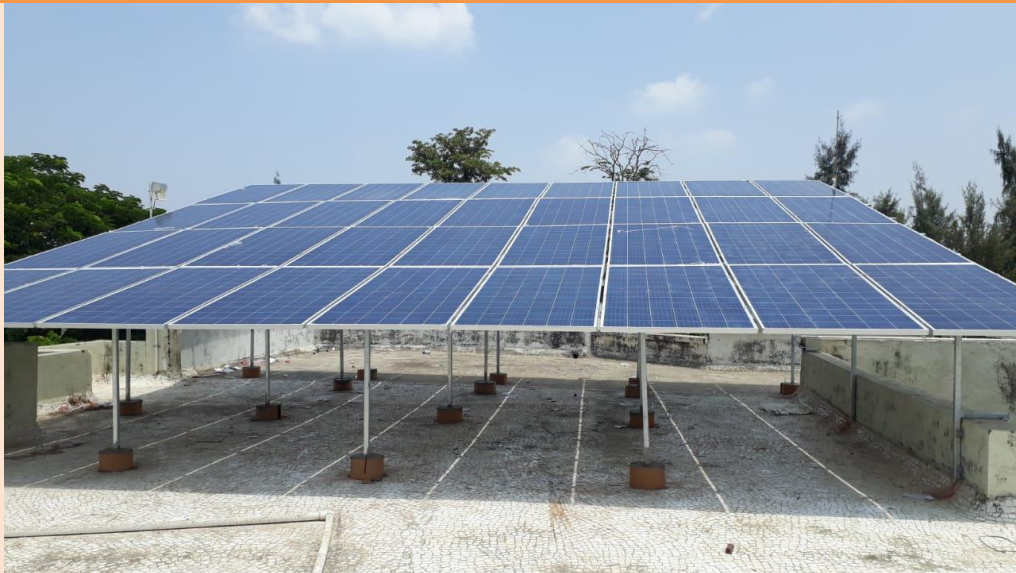
Facility of Solar panels on hostel rooftop
