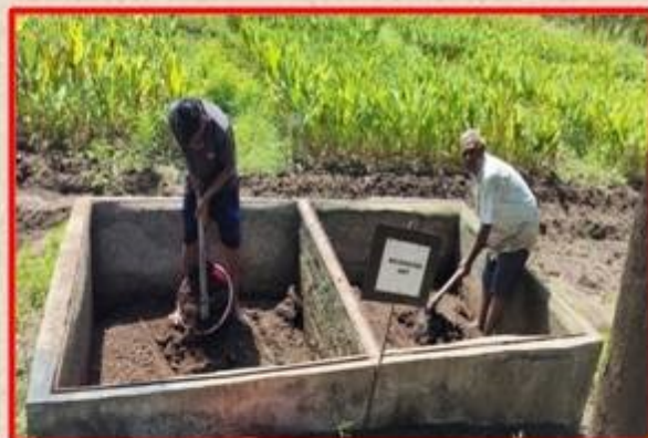
Unaerobic composting unit
